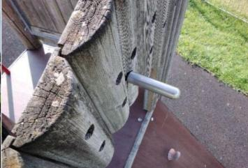
**Finding:** There is/are finger entrapment/s in the barrier and the item fails to meet the requirements of BS EN 1176 Part 1
