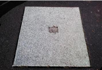
**Finding:** The wet pour has been repaired with bitmac which **Action:** Replace with a appropriate safer surface forms a hard object within the impact area
