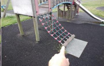
**Finding:** The net anchor forms a hard object within the impact area of the equipment in contravention of the requirements of BS EN 1176 Part 1
