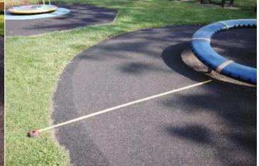
**Finding:** The surfacing dimensions are short and do not meet with the requirements of the current applicable standard
