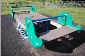
**Finding:** A number of fixing(s) have worked loose on the seat
