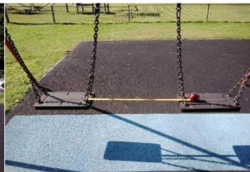
Finding: The seats are too close to each other as defined in Action: Monitor - No remedial work recommended BS EN 1176 Part 2; this is a low risk failure and no remedial action is required
