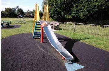
**Finding:** There are significant gaps (over 30mm) between the surface and the edging or between the joints in the surface; these are large enough for a small foot to enter
