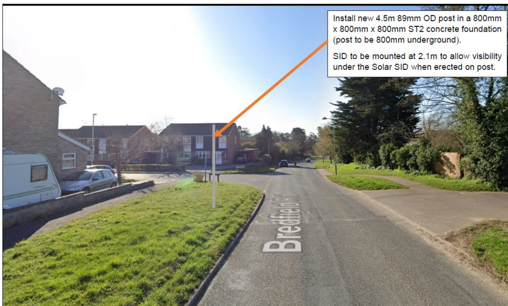
Figure 1 Site 1 - Travelling towards Woodbridge
