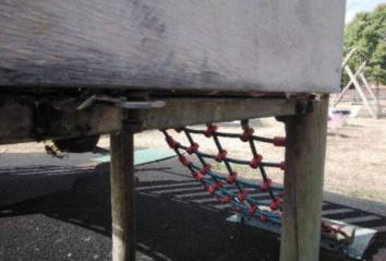
Finding: A barrier has been replaced and there protruding fixings beneath
