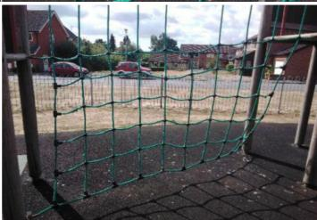
**Finding:** The ropes/nets are worn/damaged in places
