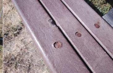
Finding: There is some evidence of fire damage to the item Action: Monitor for any further deterioration and repair as required
