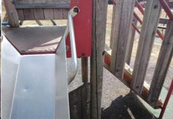
**Finding:** There are splits in the timber running through fixing **Action:** Replace all affected timber parts points and creating some instability in the structure
