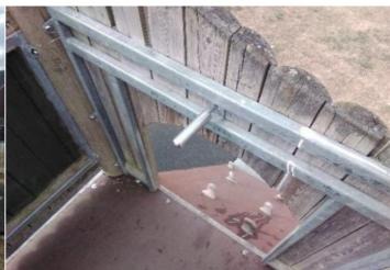
Finding: There is/are finger entrapment/s in the barrier and Action: Remove the entrapment the item fails to meet the requirements of BS EN 1176 Part 1 4.2.7.6 Entrapment of fingers
