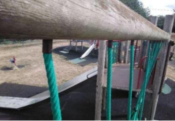
Finding: The net connections are corroding
