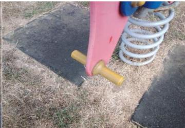
**Finding:** The end of handgrips and/or footrests have a cross **Action:** Monitor - No remedial work recommended section of less than 15cm2 and fail to meet the requirements of BS EN 1176 Part 6
