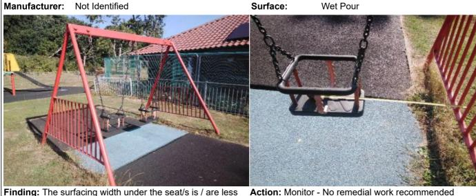
**Finding:** The surfacing width under the seat/s is / are less than 875mm when measured from the centre of the seat outwards, and fails the requirements of BS EN 1176 Part 2
