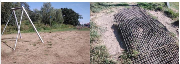
**Finding:** The edges of the grass mat surface have not been **Action:** Tuck in edges of grass mat to remove trip hazards installed in accordance with the API Code of Practice
