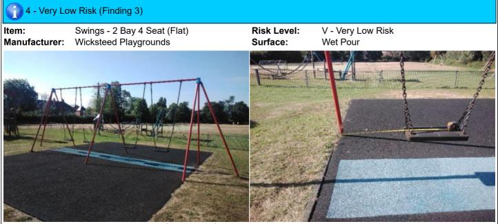
**Finding:** The seats are too close to the frame as defined in **Action:** Monitor - No remedial work recommended BS EN 1176 Part 2; this is a low risk failure and no remedial action is required
