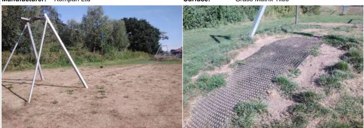
**Finding:** The grass has eroded within the impact area of the **Action:** Reinstate the grass or provide an all weather equipment and may not provide the necessary impact attenuating properties for the equipment fall height; the surface may also be slippery in wet weather
