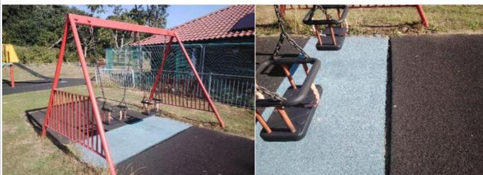
**Finding:** There are significant gaps (over 30mm) between the surface and the edging or between the joints in the surface; these are large enough for a small foot to enter
