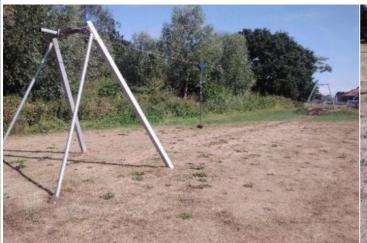
**Finding:** The height of the seat is less than 350mm when loaded and does not meet the requirements of BS EN 1176 ground level when loaded with 69.5kg Part 4
