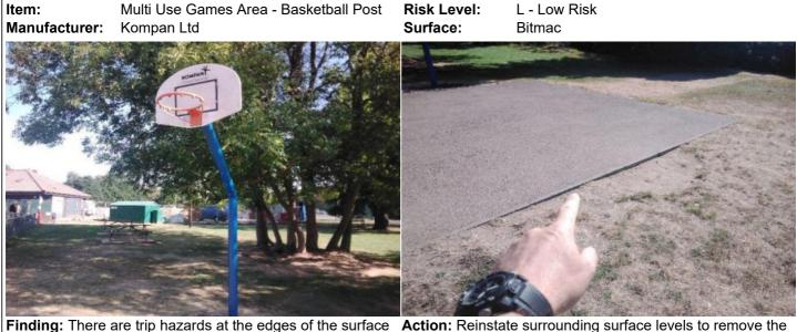
Finding: There are trip hazards at the edges of the surface trip points
