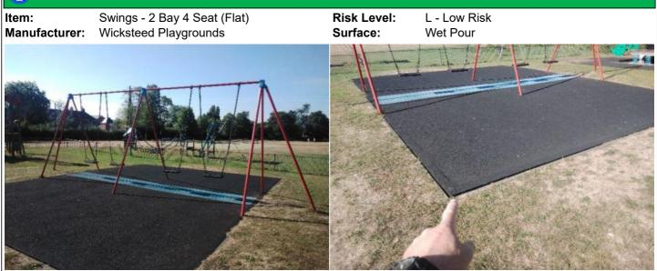
**Finding:** The surface is lifting at the edges and creating trip **Action:** Repair perimeter of surfacing to remove trip points
