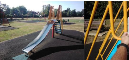
Finding: The item fails to meet the requirements of BS EN Action: Monitor - No remedial work recommended 1176 Part 1 4.2.7.2 head and neck entrapment in the barriers and/or steps
