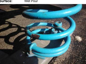
Finding: The paintwork on this item has been damaged or Action: Treat any rusting components and repaint worn exposing the metal underneath which is rusting
