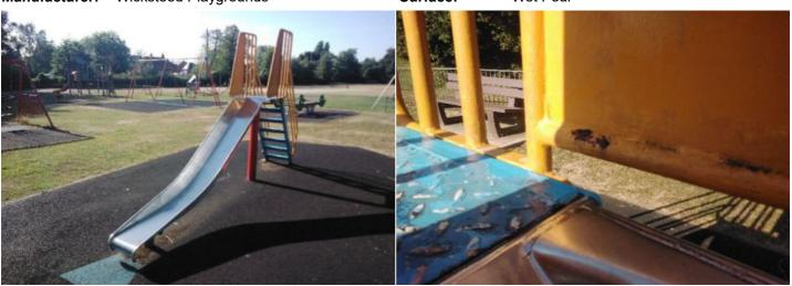
Finding: The paintwork on this item has been damaged or Action: Treat any rusting components and repaint worn exposing the metal underneath which is rusting
