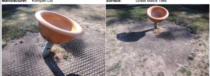
**Finding:** The grass mats are silted up, the soil is compacted **Action:** Reinstate as required and the area will become very slippery when the soil is wet.
