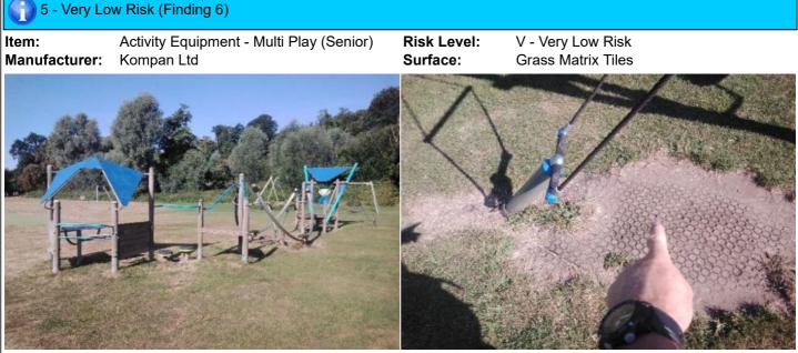
**Finding:** Fixing Pins have been installed in the impact areas **Action:** Remove pins from impact areas of the grass mats
