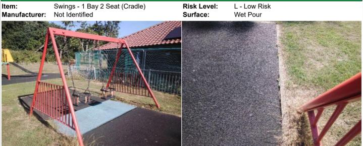
**Finding:** There are gaps opening between the surfacing and **Action:** Monitor for any further deterioration and repair as the edging surround or between the joints in the surfacing required
