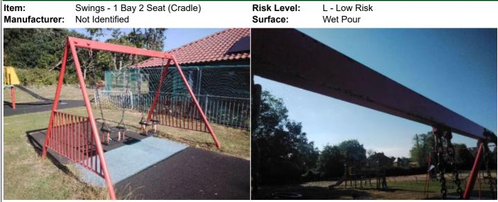
**Finding:** The paintwork on this item has been damaged or worn exposing the metal underneath which is rusting
