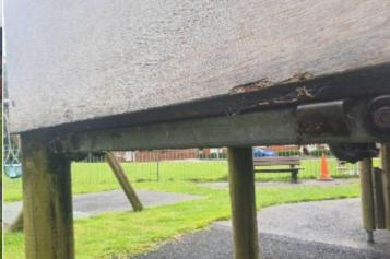
**Finding:** A barrier has been replaced and there are metal brackets remaining creating sharp edges
