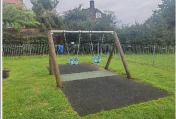
**Finding:** There is algae or moss on the surface of the equipment which can lead to the onset of rot
