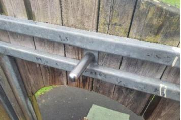
**Finding:** There is/are finger entrapment/s in the barrier due **Action:** Provide missing fixings to remove entrapment to missing fixings and the item fails to meet the requirements of BS EN 1176 Part 1 4.2.7.6 Entrapment of fingers
