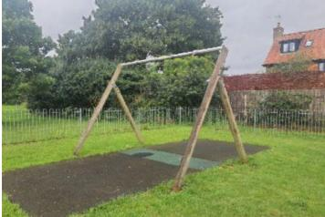
**Finding:** There are areas or parts of the timber on the structure that have rotted (Risk assessment has been lowered due to there being no swings attached)
