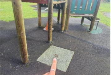
**Finding:** The wet pour has been repaired with bitmac which **Action:** Replace with a appropriate safer surface forms a hard object within the impact area
