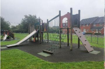
**Finding:** The inspector has some concerns about the internal condition of the timber and was unable to verify the structural integrity without further testing. We recommend a Resi-PD survey to establish the condition of the timber at it's core. **Action:** Contact th further information structural integrity without further testing. We recommend a Resi-PD survey to establish the condition of the timber at it's core.
