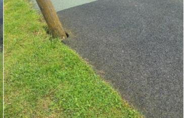
**Finding:** The surface is lifting at the edges and creating trip **Action:** Repair perimeter of surfacing to remove trip points points
