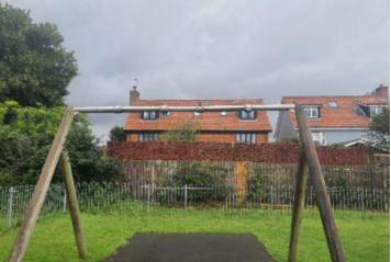
**Finding:** The seat(s) and suspension were missing at the time of inspection and the inspector was unable to make a full compliance assessment
