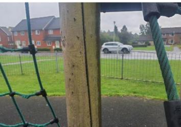
**Finding:** The timber has a number of splits/shakes or air cracks and this may affect the stability or allow water ingress fixing points of the structure and/or cause any instability which will accelerate the rotting process
