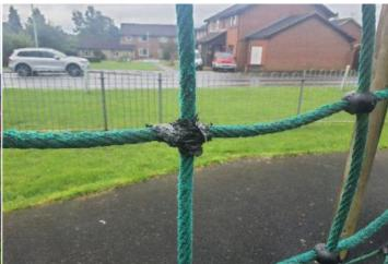
Finding: The ropes on this item have been taped and we are unable to fully assess the condition of the rope, ensure no wire strands are broken beneath the tape
