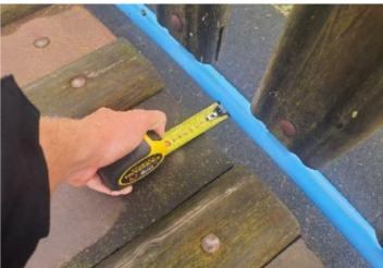
Finding: There are gaps in excess of 30mm in the direction Action: Monitor - no remedial action recommended of travel creating foot entrapment/s in contravention of BS
