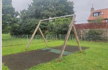
Finding: Parts of the timber are rough or splintered
